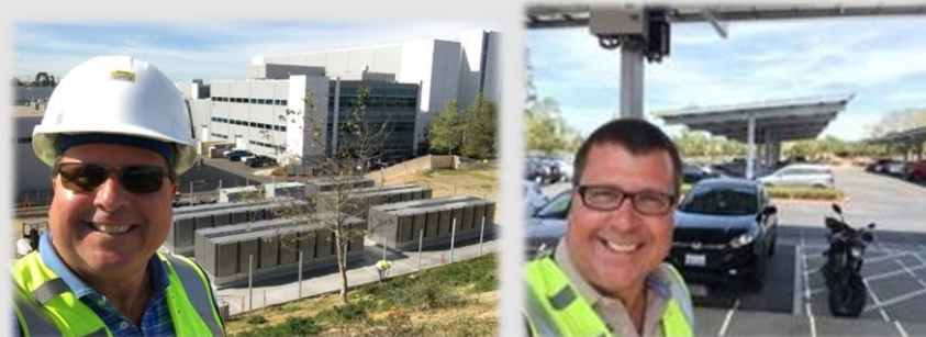
2.5 MW Fuel Cells and 3.8 MW Solar Arrays.
